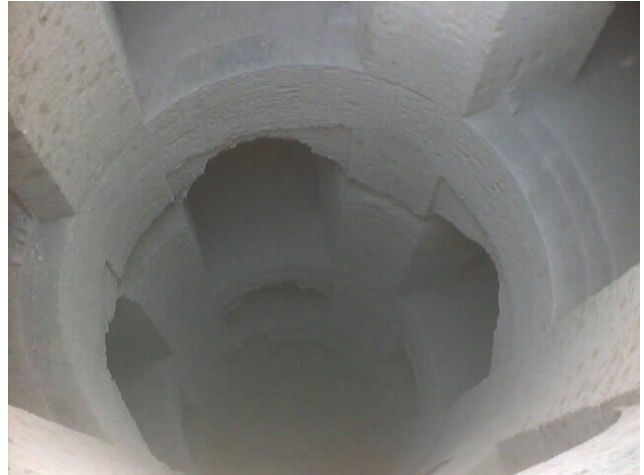
Central shaft in the Palace
