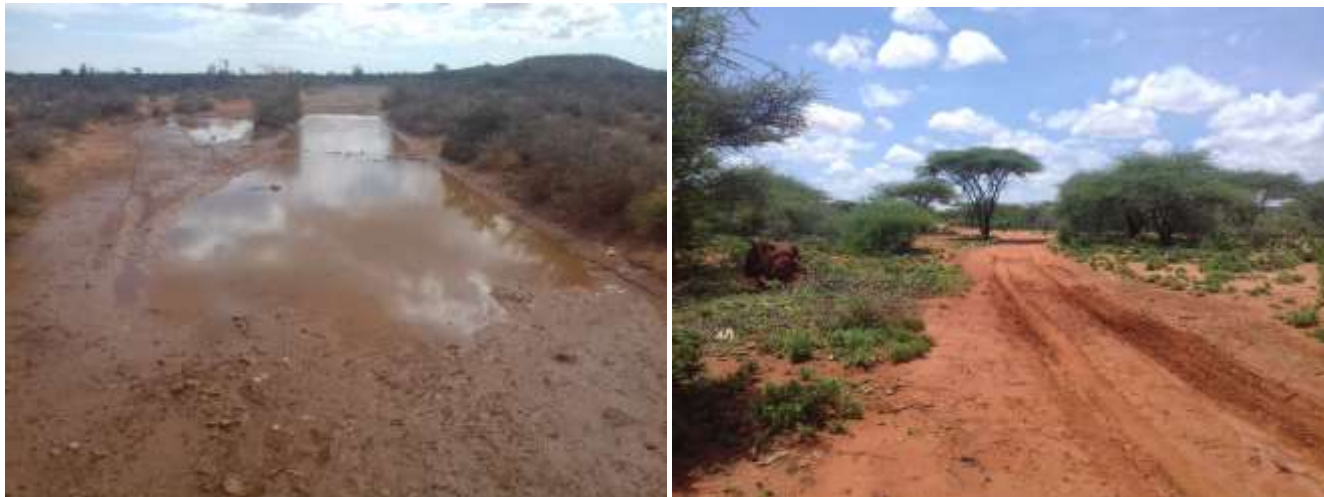
The road to Buuhoodle: section near the beginning, and past half-way.
